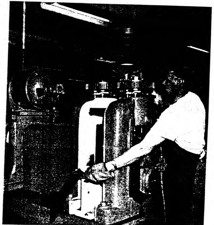
NO. 3—After specified amounts of 24-kt. gold, silver and copper have been melted and cast into ingots of 14-kt. gold (see cover picture), the ingots are put through a rolling mill to reduce them from a thickness of 1/2 inch to the normal working thickness of 1/20,000th of an inch. The employee is Paul Lake.
